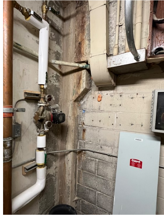
Photo 14: Vertical crack propagating up length of column. This column is adjacent to Room 1030A and the beam in question.
